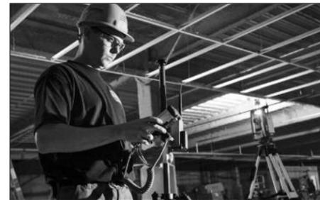
**HIGH TECH IN THE FIELD.** A plumber uses a Total Station Layout Trimble GPS device on a Cannistraro project.
